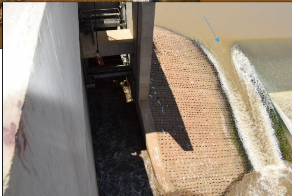
Lower Thukela Bulk Water Supply Scheme weir; eelway
